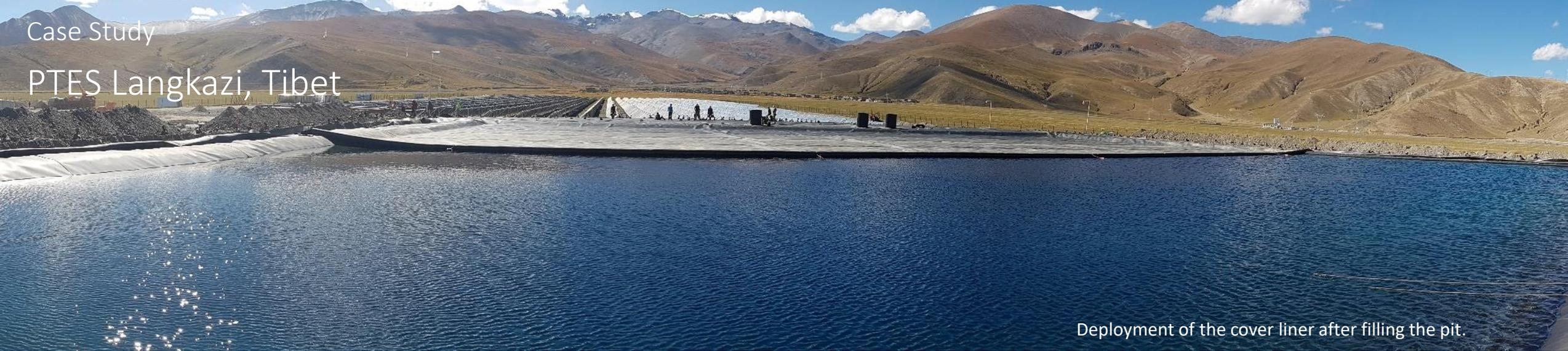
Deployment of the cover liner after filling the pit.
