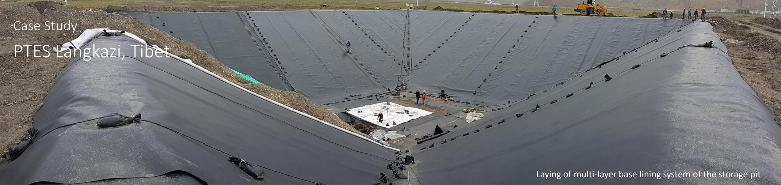
Laying of multi-layer base lining system of the storage pit
