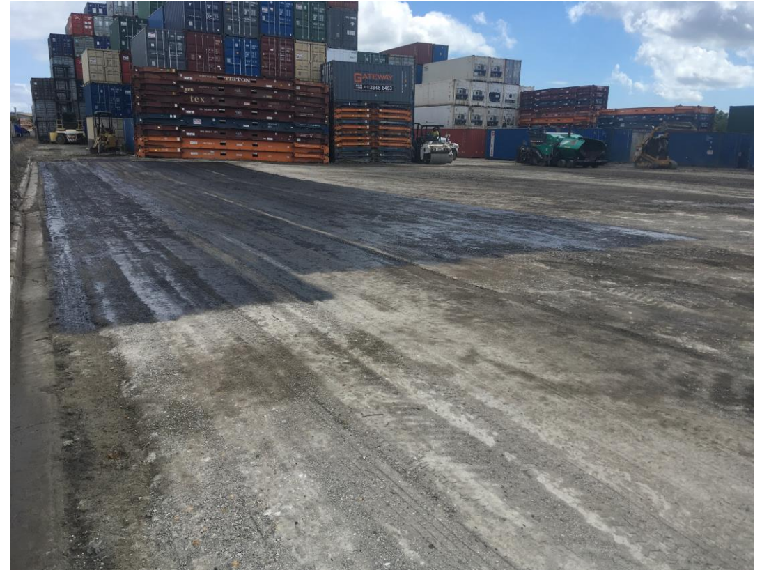
Figure 2. CTB Pavement – AMC-0 Priming
