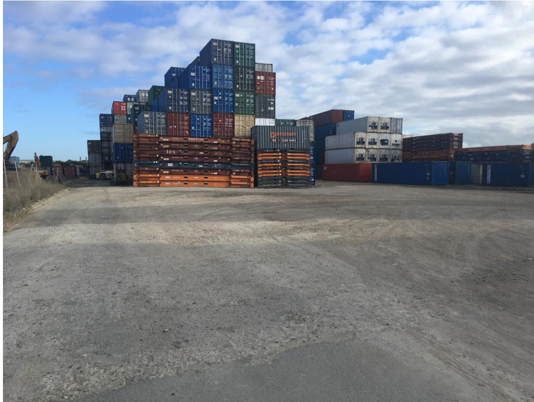
Figure 1. CTB Pavement – Prior to Works
