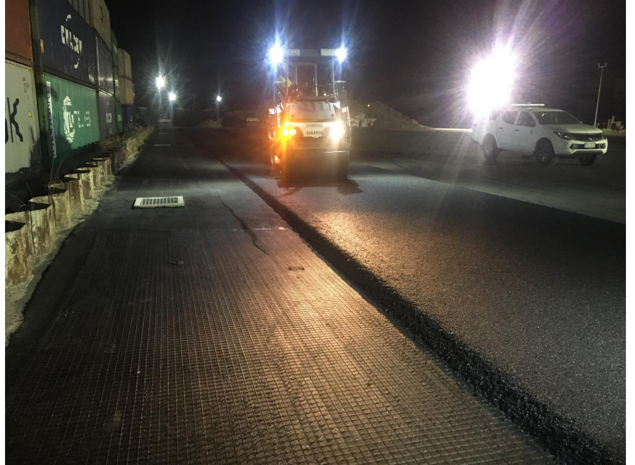
Figure 8. EME2 - Under Construction
