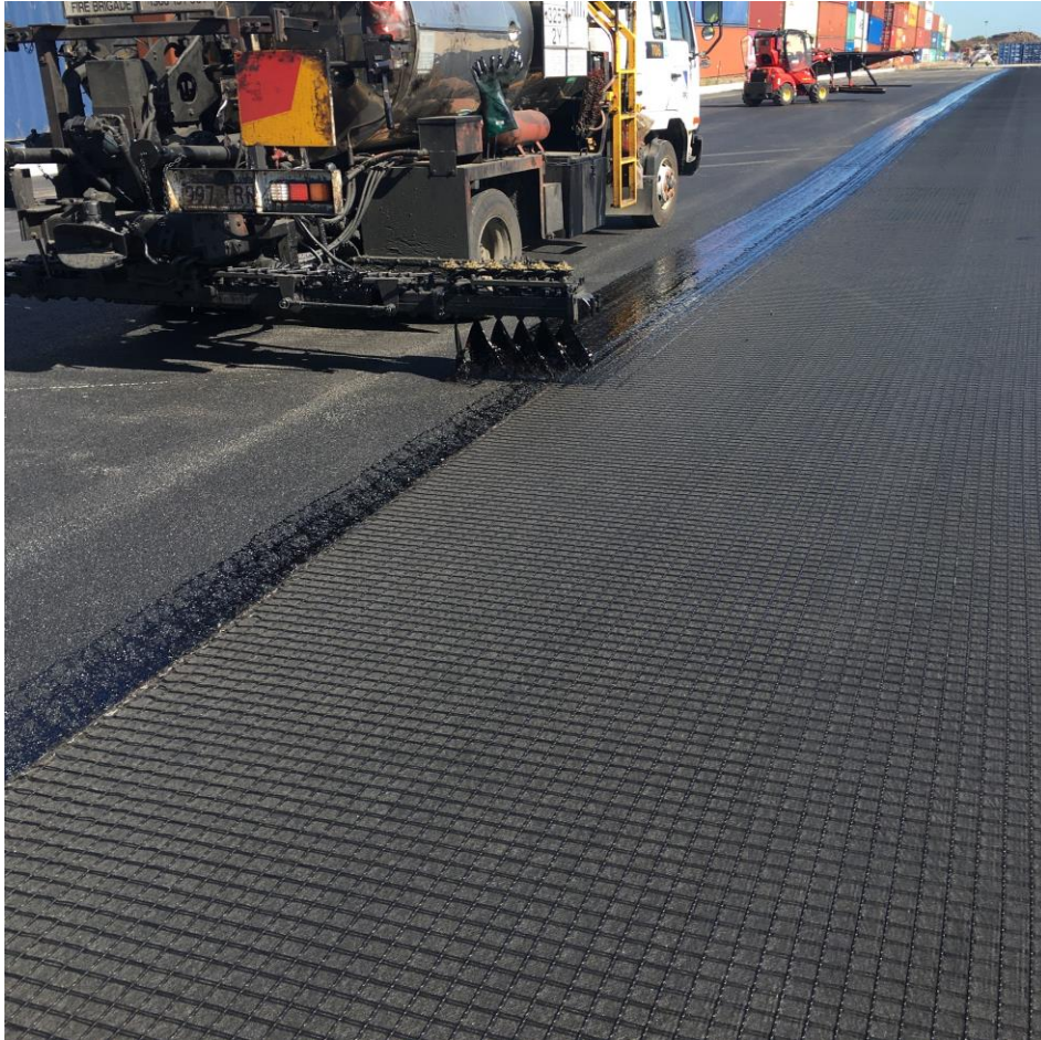
Figure 5. Tack Coat and HaTelit C
